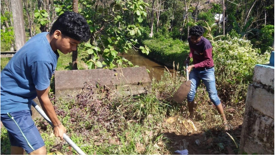
NSS VOLUNTEERS CONSTRUCTING DRAINAGE AT MELUKAVU GRAMAPANCHAYATH
